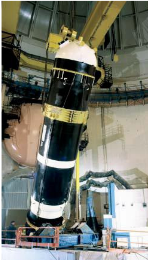
Figure 9: The pressurizer
