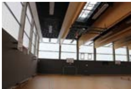
Fig. 1. Example of a building with granular aerogel filled PC panels.
