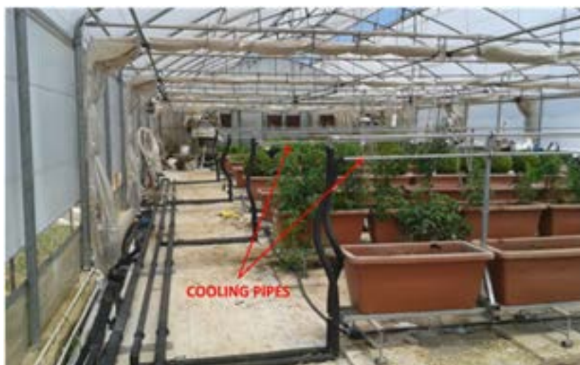
Figure 1. The inside of the experimental greenhouse and the cooling distributing system.
